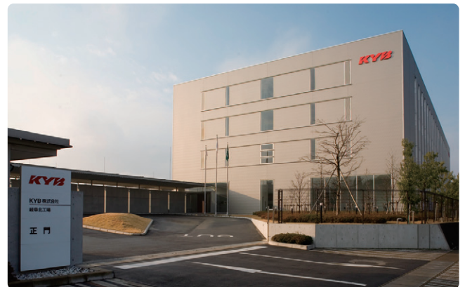
Gifu North Plant
