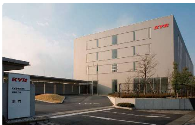
Gifu North Plant
